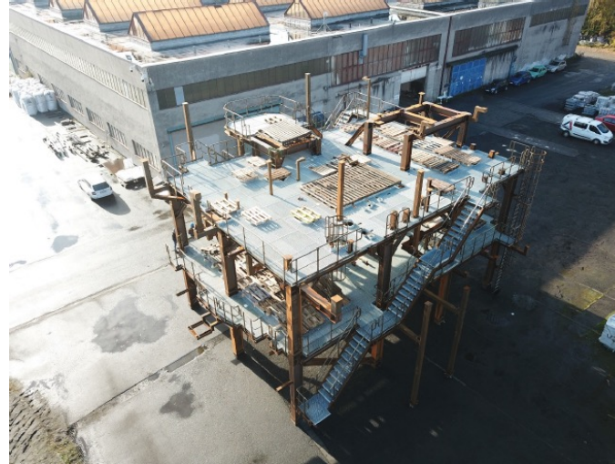
Module preassembled in Lithuania
